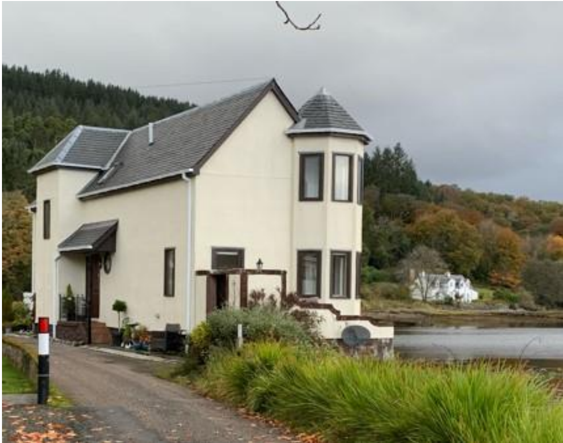
Lochside -There is no precedent in the area for the stair tower or the viewing tower. Ridge height is understood to be higher than the original property The Old Manse is in background
