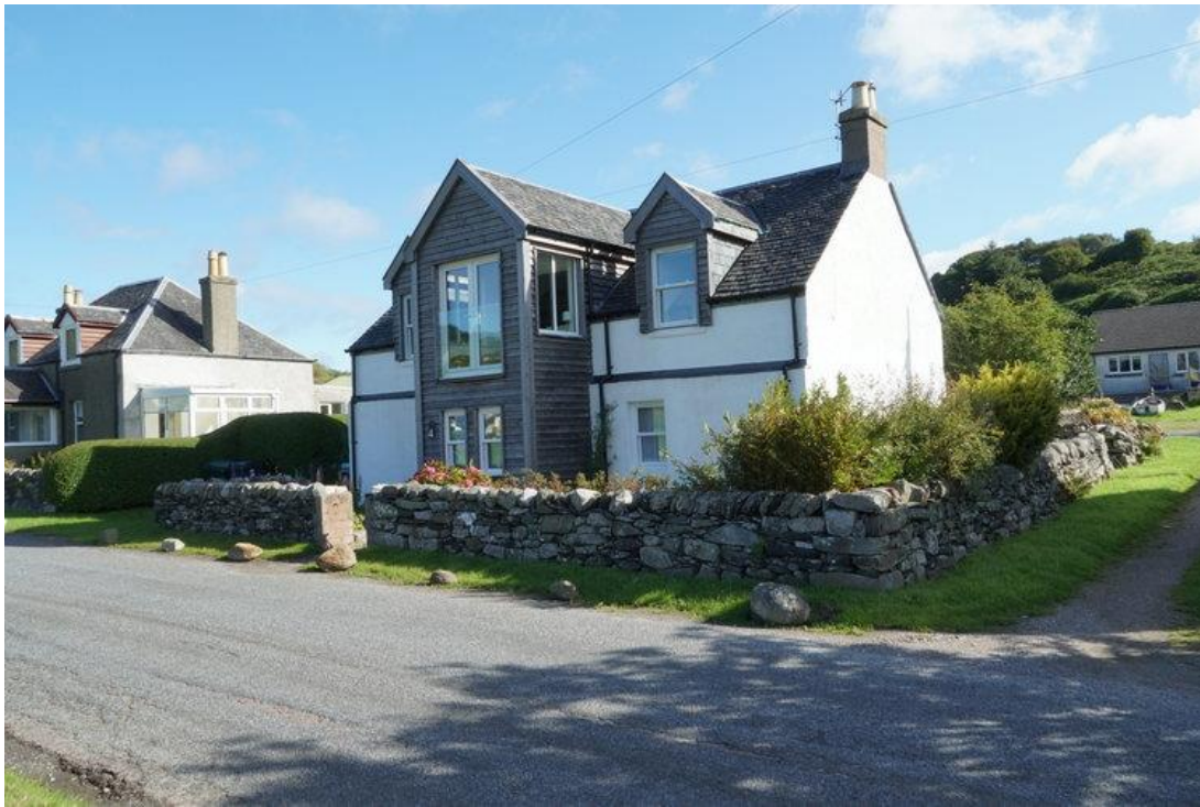
House extension at Tayvallich, shows a larch clad extension, with a broken eaves line.
